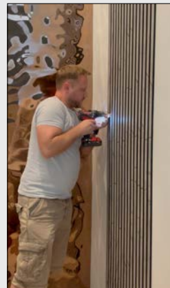
When installing without adhesive, 8 to 10 screws are recommended.
